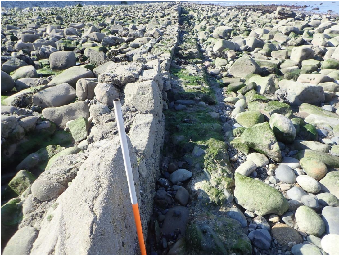
Plate 22: View looking north at base of retaining wall with external layer that might be an exposed plinth or an additional basal layer. Position of image indicated on Figure 4.
