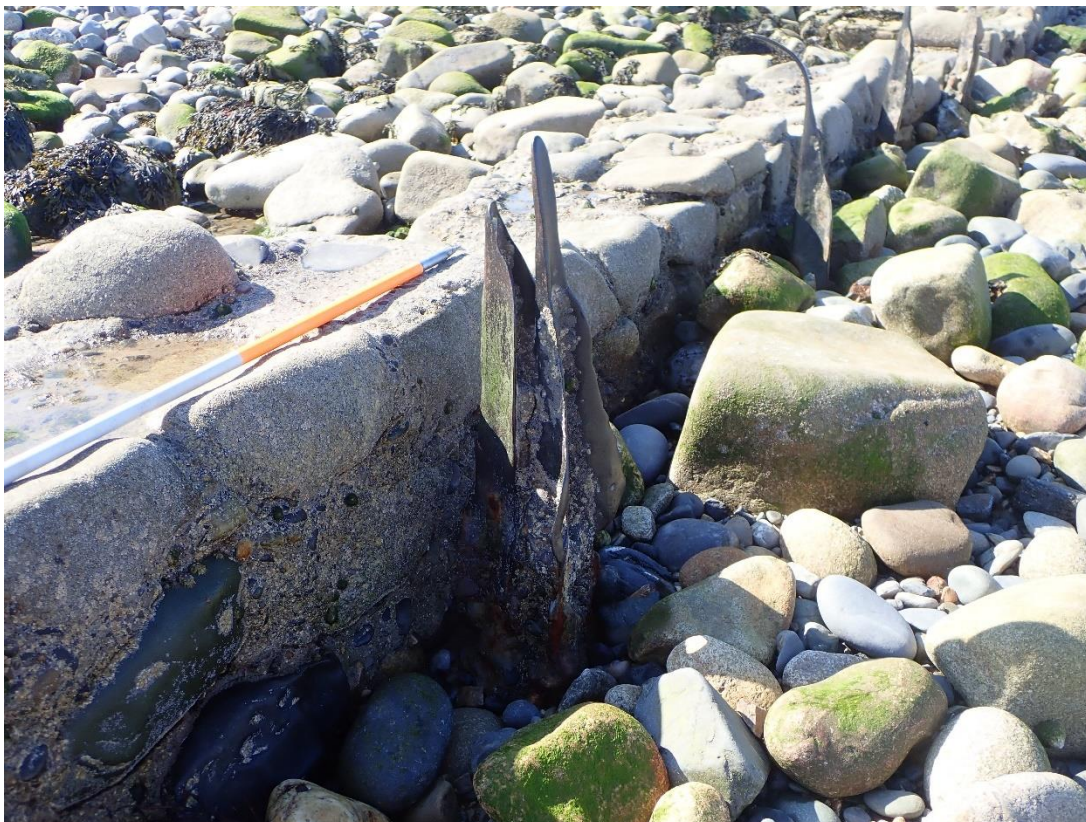
Plate 34: View of historic sheet piling that runs along exterior of railway retaining wall to the south of the project area. The steel piles are heavily eroded by coastal processes.
