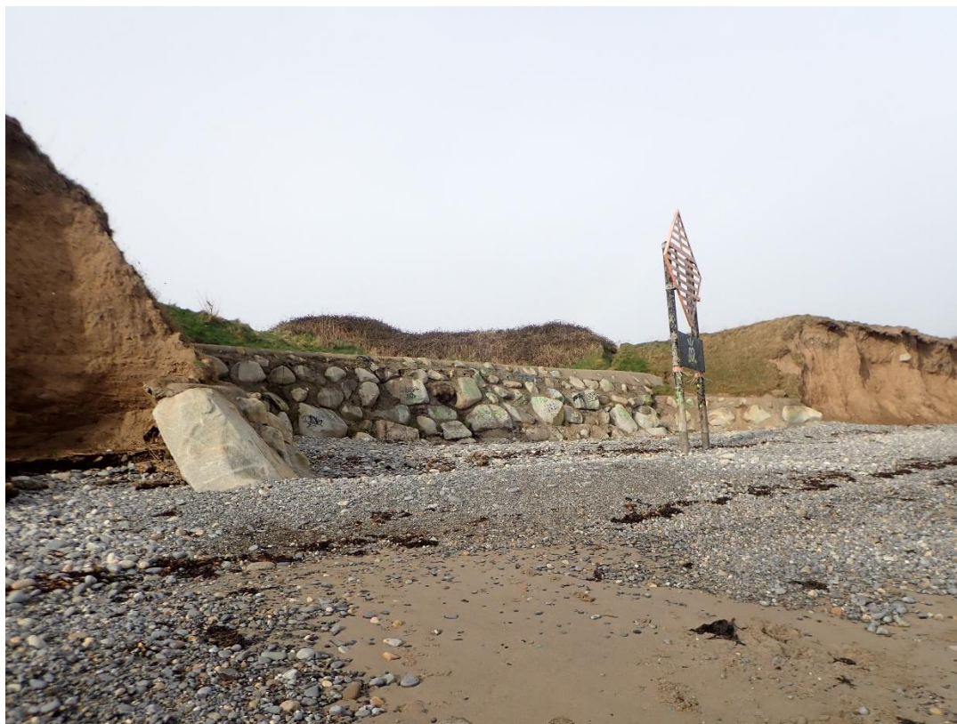
Plate 37: Landfall location of the Shanganagh Long Sea outfall. The works have cut away the sea cliff and inserted a mortated boulder barrier. The cut is clearly visible on Figure 9, as is the back-filled trench that accommodates the sewer pipe extending out to sea.
