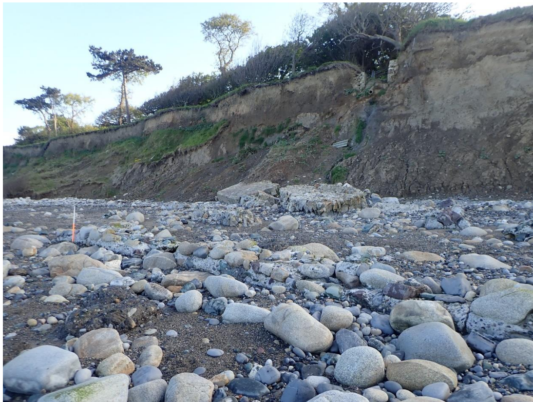
Plate 31: View looking south at the line of mortared stone that is the base of the railway retaining wall that continued north from the Clontra House underpass. The ruined underpass is visible at the cliff-top.
