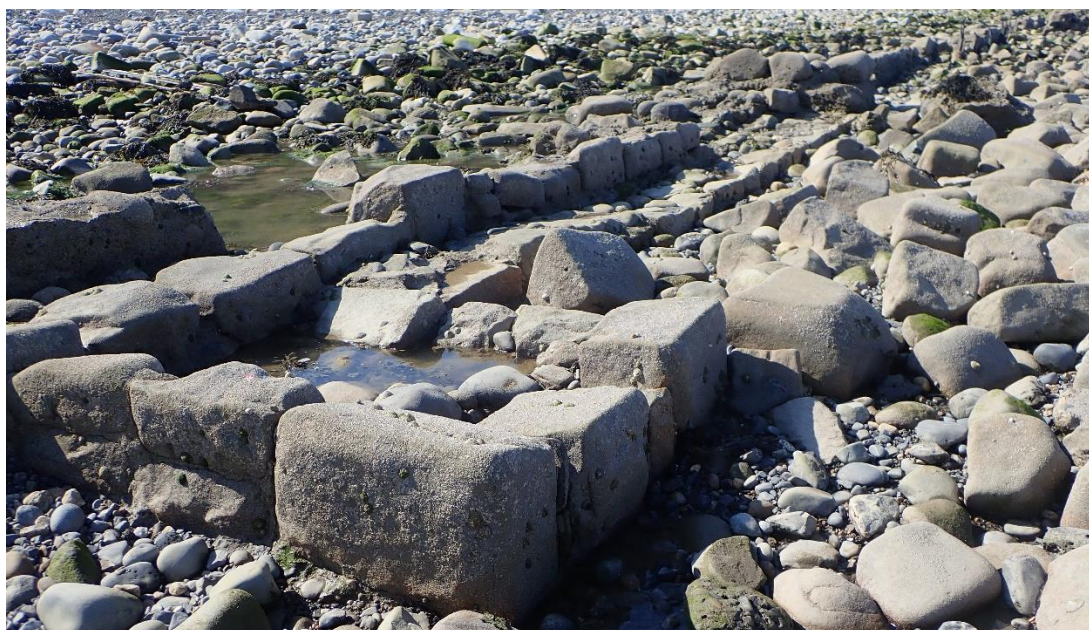
Plate 14: Example of stone buttress that forms part of the retaining wall south of the project area.
