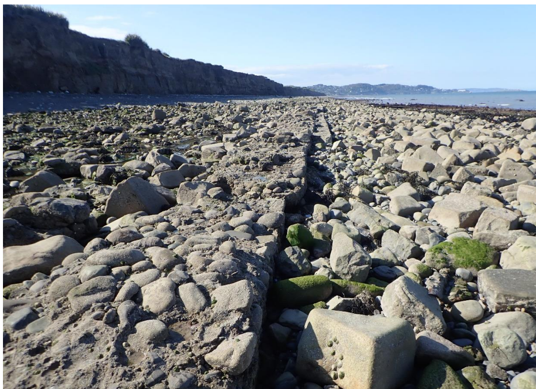
Plate 18: View looking north at base of retaining wall showing intact wall core. Position of image indicated on Figure 4.
