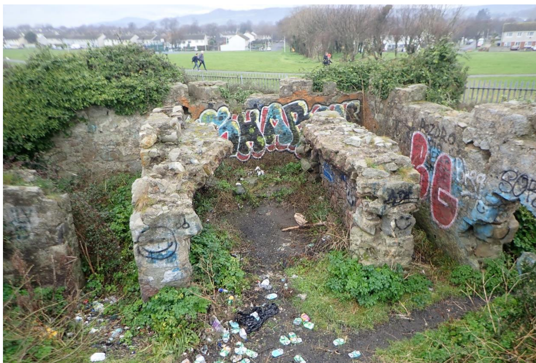
Plate 11: View looking west at squat building that supported a brick barrel vault, within the Battery enclosing wall.
