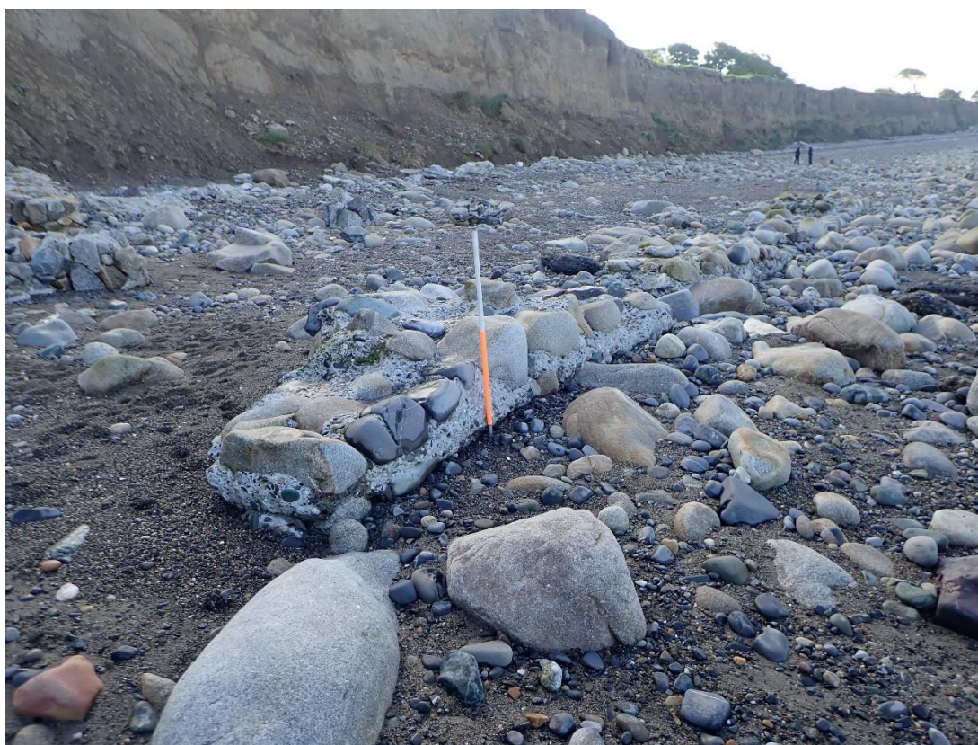
Plate 30: View looking North-northwest at the line of mortared stone that is the base of the railway retaining wall that continued north from the Clontra House underpass.
