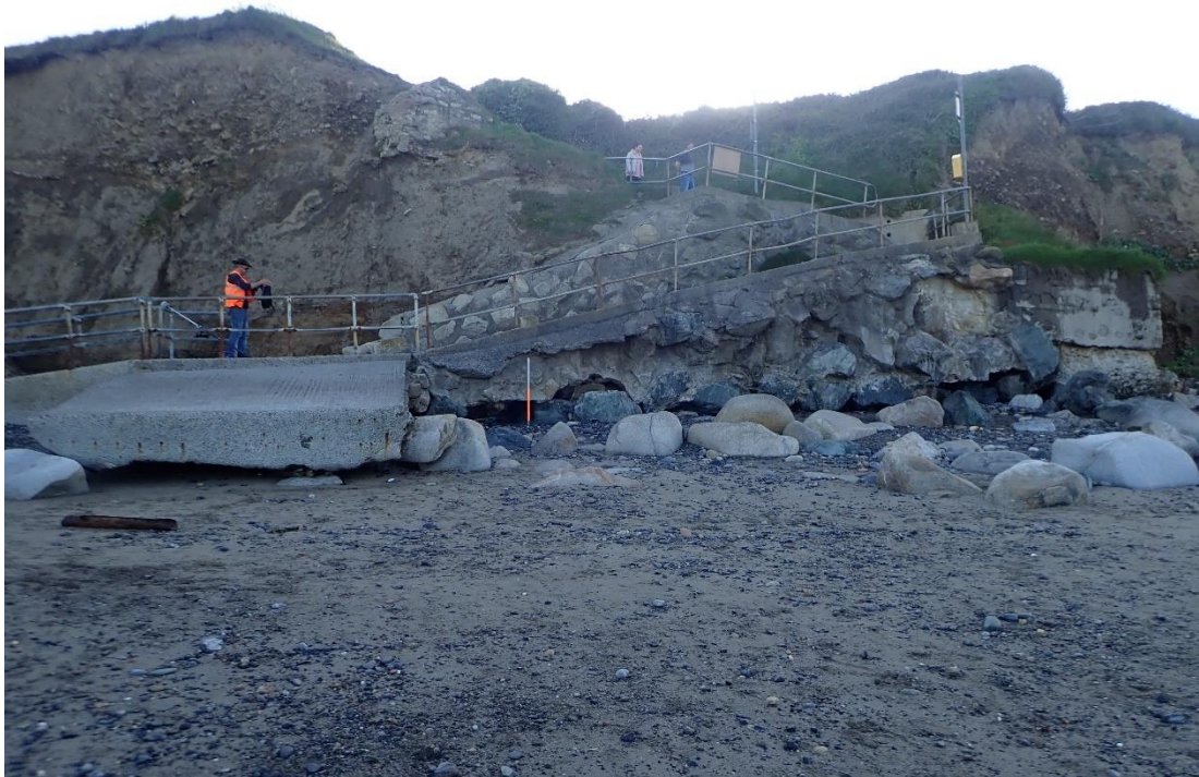
Plate 27: View looking inland from the foreshore towards the reinforced access to Shanganagh beach today. Note the modern concrete works are undercut by coastal erosion.
