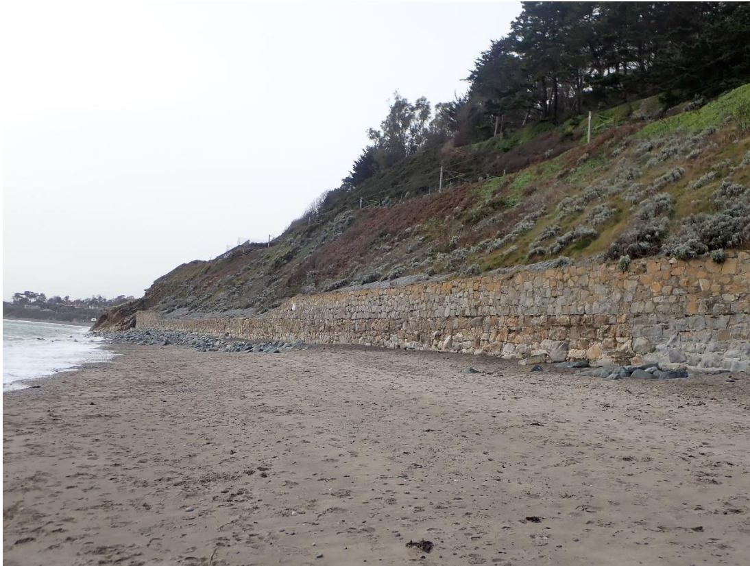
Plate 16: View of railway retaining wall at White Rock beach north of the project area. The granite-built wall retains a sloped embankment on top of which the railway line runs. It offers a comparator to what might have existed originally in Shanganagh.
